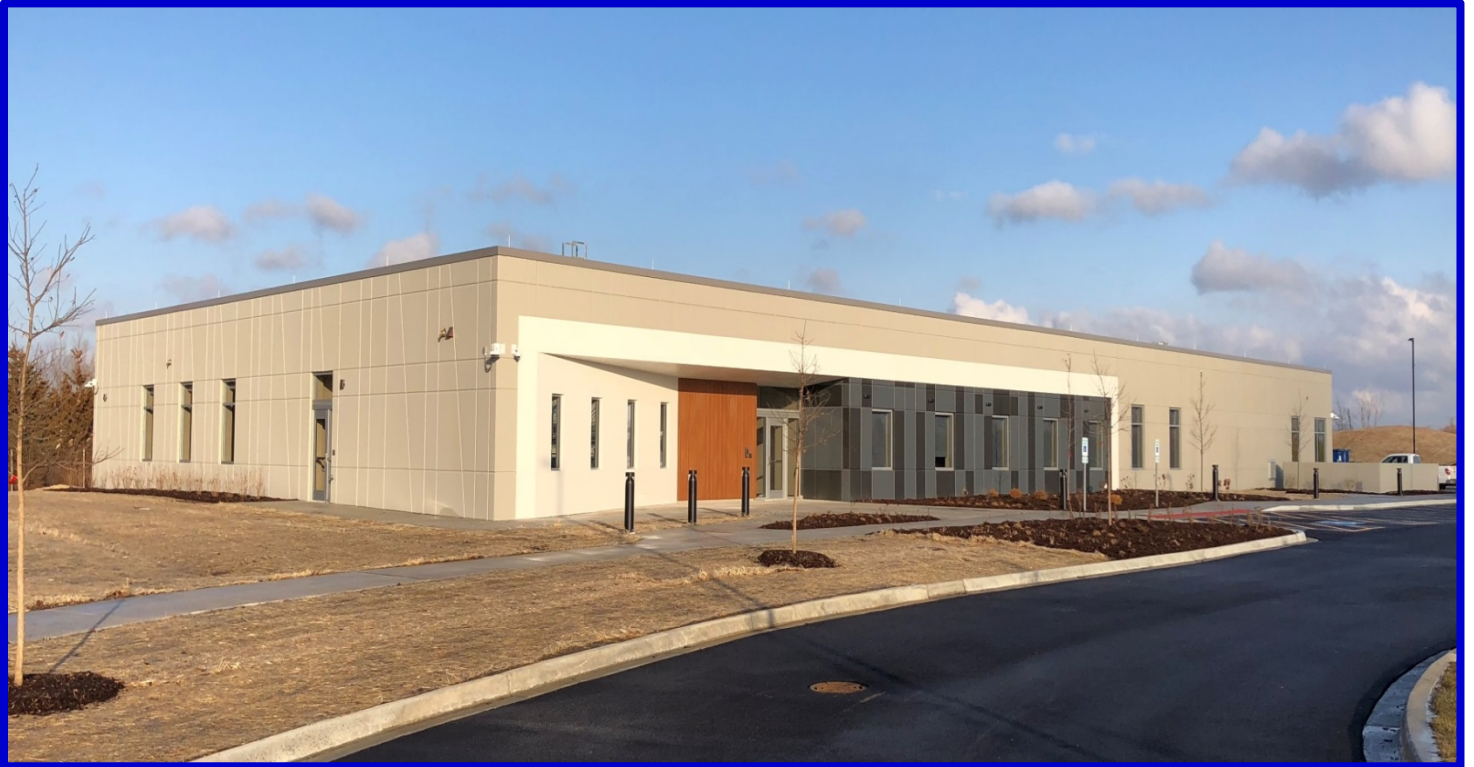
New Addison Consolidated Dispatch Center 2018
